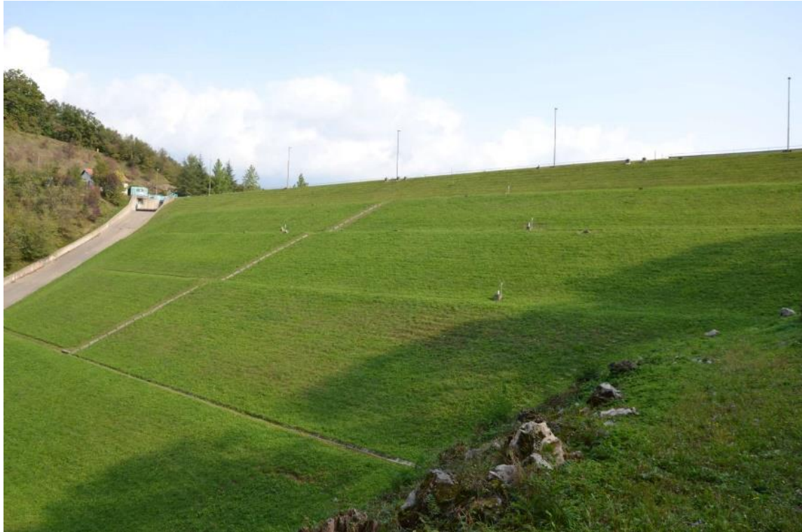
Figure 1: The downstream view of the dam.
