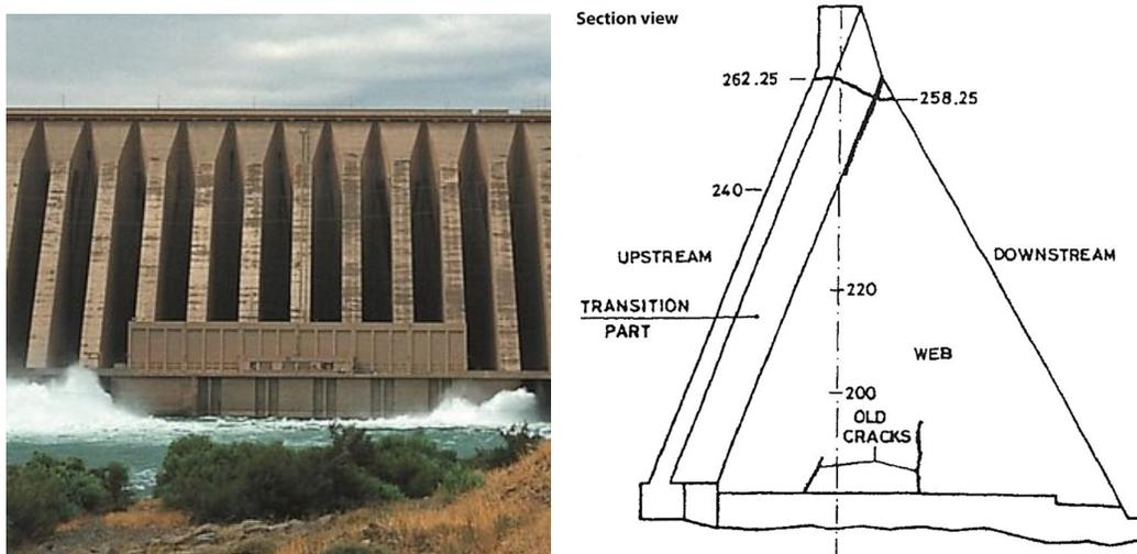
Figure 15 – The downstream view of the Sefid Rud Dam (left) and cracks after the earthquake (right).
