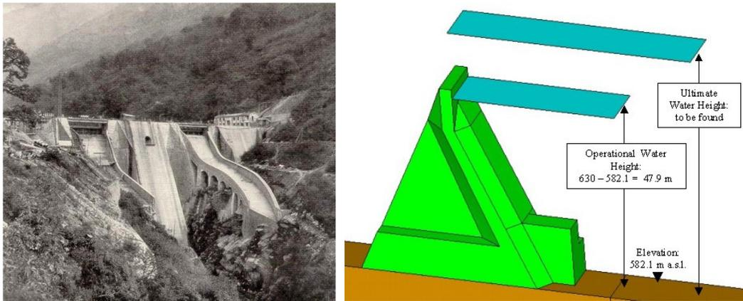
Figure 11 – Downstream view of Poglia Dam (left) and geometry of the main block and water heights to be considered (right).
